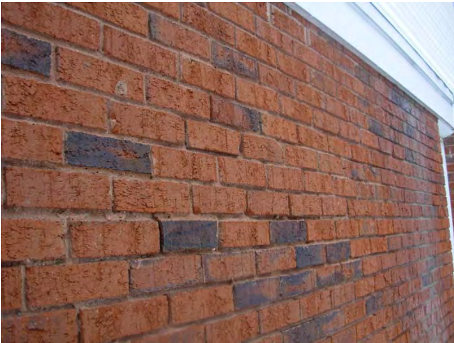
5. Minimal mortar deterioration at some gable end walls
