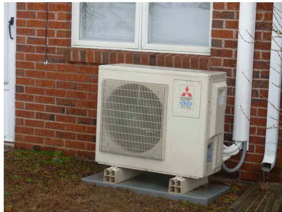
16. Heat pump HVAC system exterior condensers, typical
