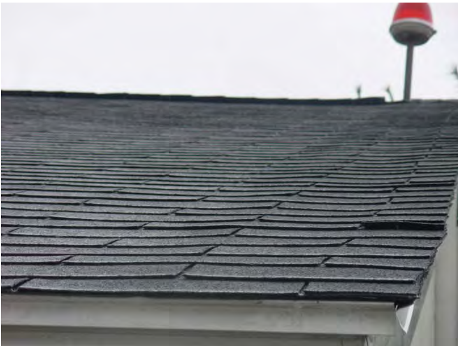
7. Spot lifting roofing shingles
