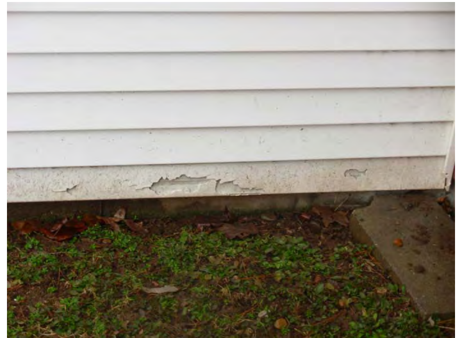
6. Spot vinyl siding damage
